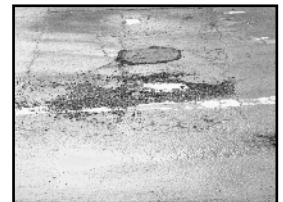
Repaired potholes in Chichester Road
